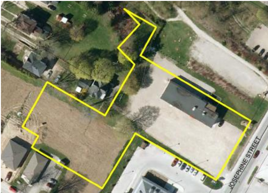
Figure 1. Subject Parcel – Air Photo (property outlined in yellow)
