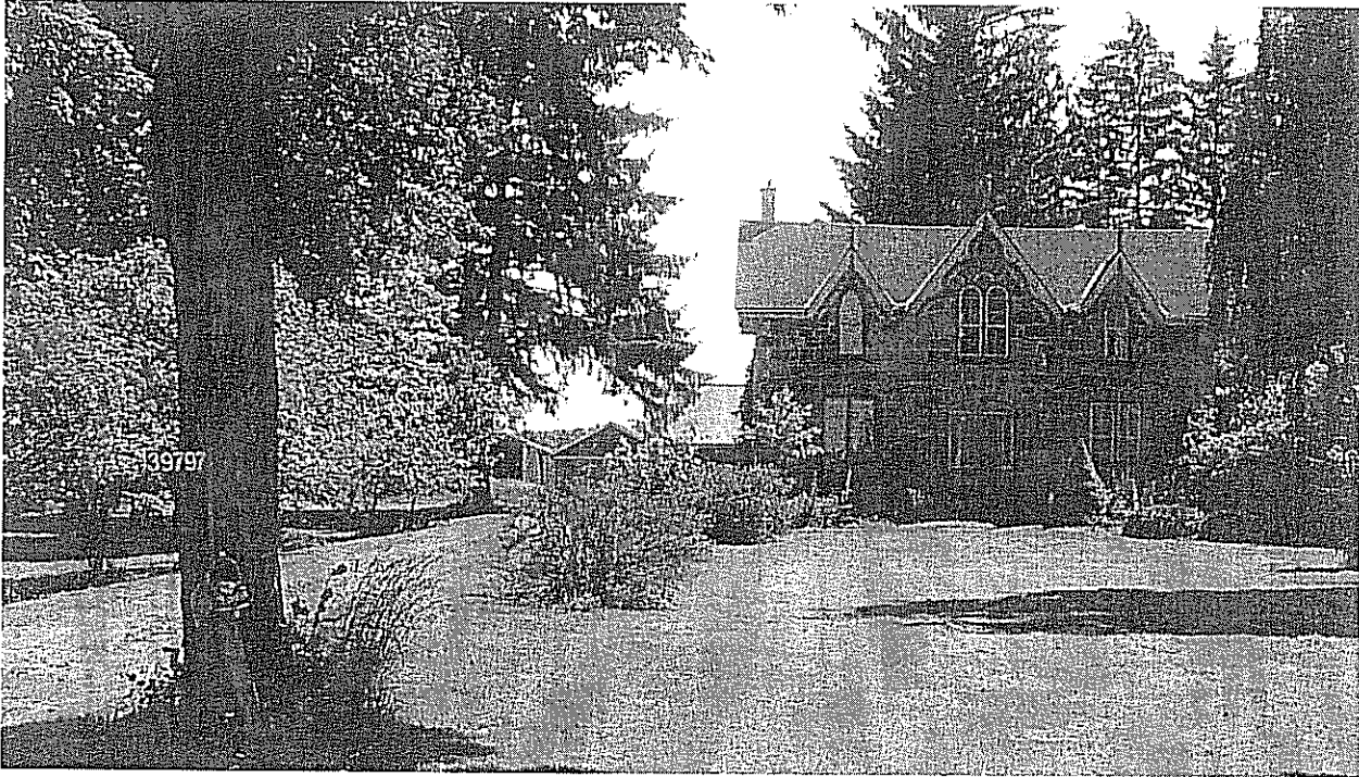
Standing on Belfast Road, looking at the severed parcel
