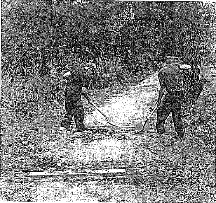
Terry and Mike installing the erosion control strips
